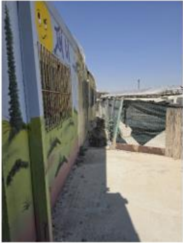
A disintegrating fence at Al-Azazma A
