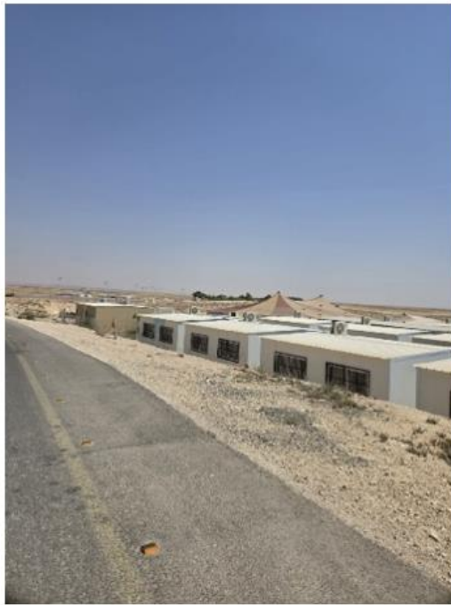
The classroom compound at Wadi al-Na'am High School, exposed to the road
